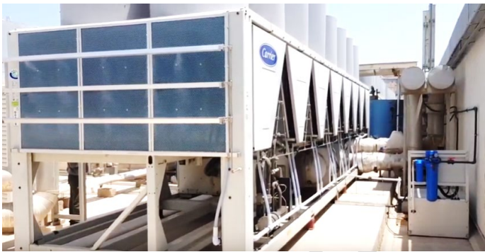
(Picture No.2 Chiller equipped with “Smart Cooling™” system)
