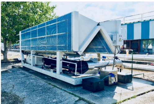
(Picture No.2 Chiller equipped with “Smart Cooling™”)
