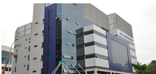
Communication Data center India, Pune
