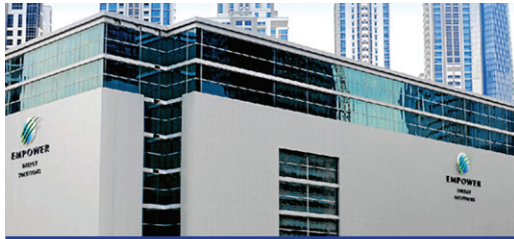
EM Power district cooling plant Dubai, UAE
