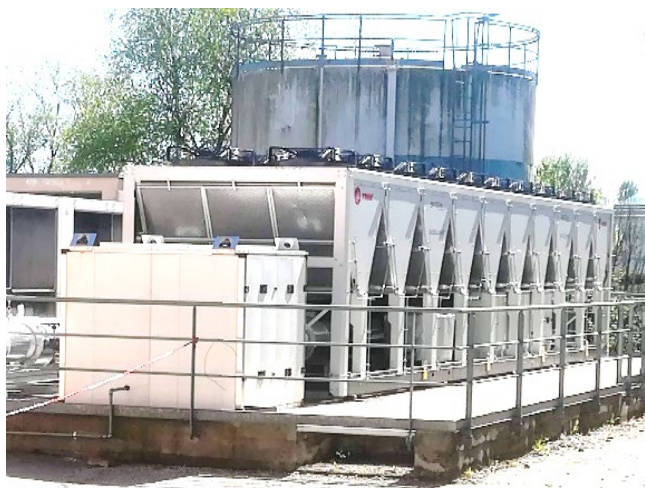
(Picture No.2 Chiller equipped with “Smart Cooling™” system)
