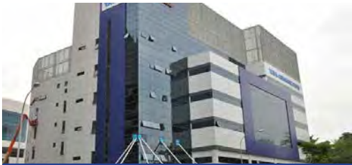
Communication Data Center-Pune, India
