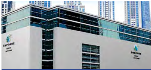
EMPOWER district cooling plant Dubai, Dubai UAE
