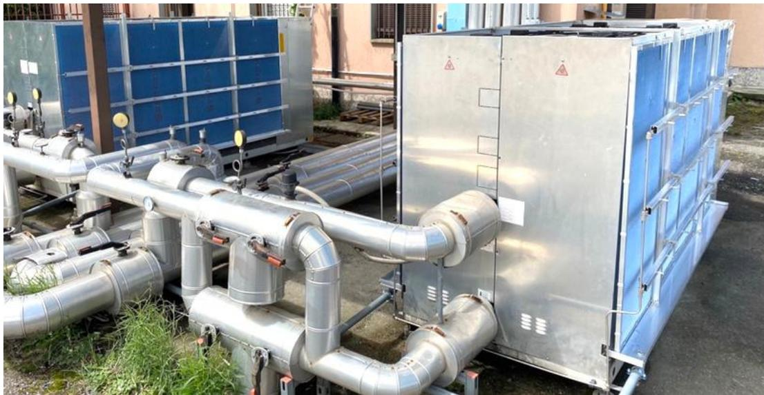
Picture 2; Chiller with **Smart Cooling™** system
